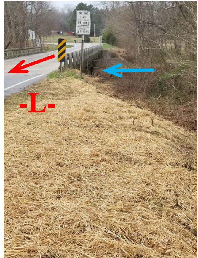
Standing at End Bent 2 and looking West
