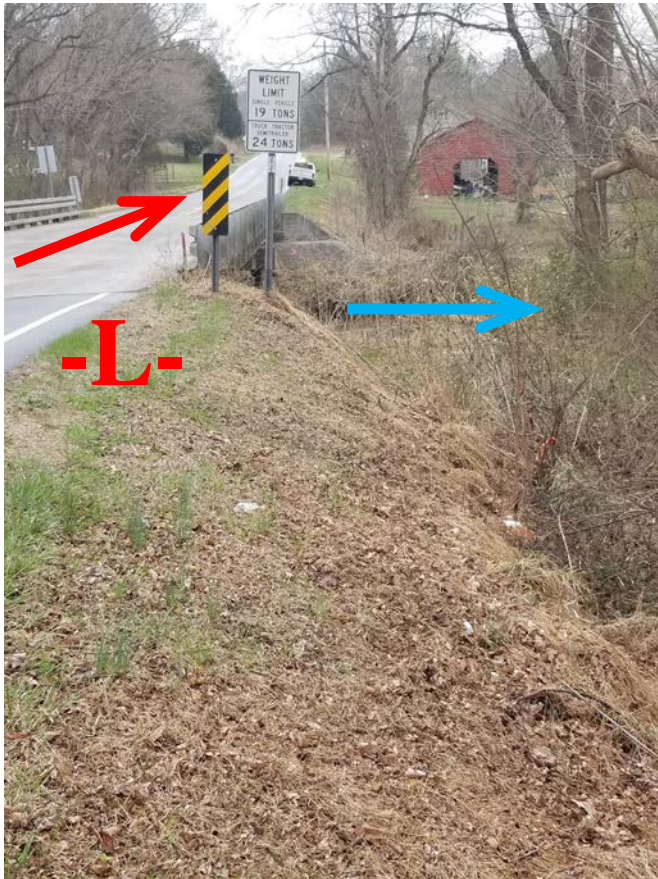
Standing at End Bent 1 and looking East
